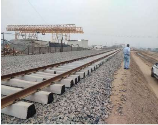
Pirthala Railway Yard (start point of alignment)
