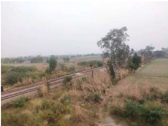
Delhi Rohtak Railway line
