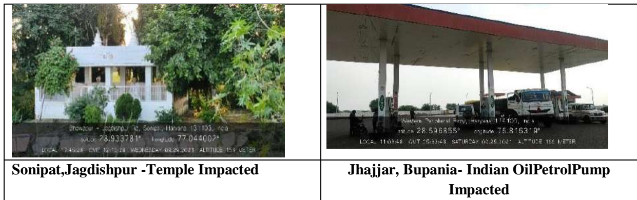
Figure 1-4: Photographs of the structures Impacted
